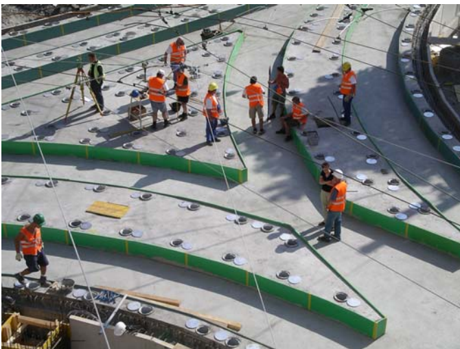
Fig. 14 Lifting and adjustment of the track slab
