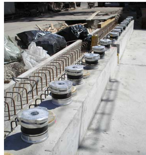
Fig. 15 Spring units prepared for installation
