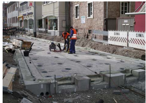
Fig. 8. Lifting of the concrete slab
