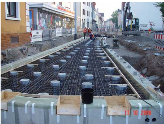
Fig. 7. Slab construction, embedded spring housings
