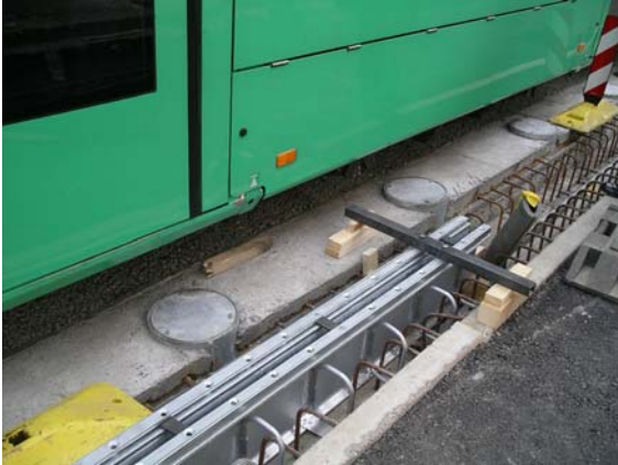
Fig. 11 Installation of the elastic joint sealing during tram operation Fig. 12 Detail [3]
