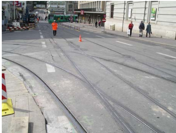
Fig. 9 Tram track system in front of the concert hall before replacement
